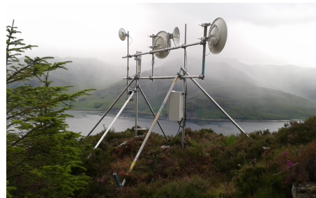
Figure 4: A basic relay
