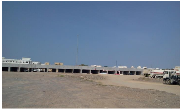
Culverts between Al-Hail north and south in Sultan Qaboos Road
