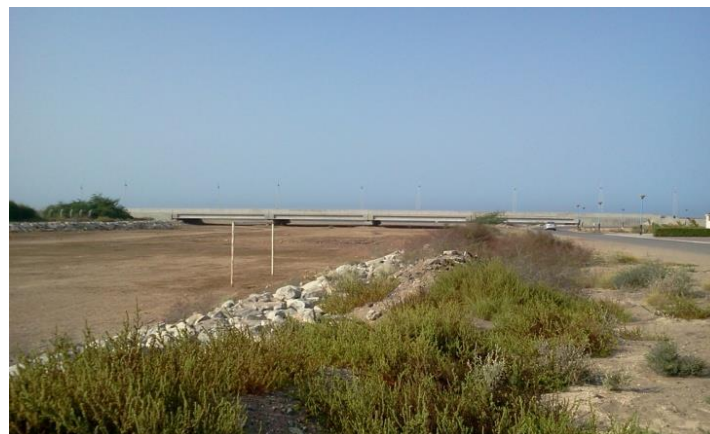
Culverts near the sea.
