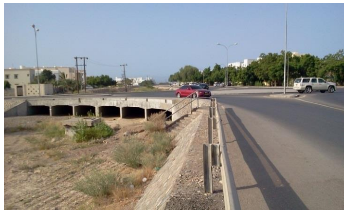
Culverts in the middle of Wadi Alkhurys
