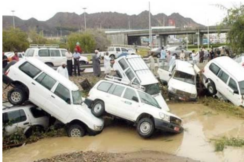
Figure 5.2: Culvert problems in Muscat (2007)
