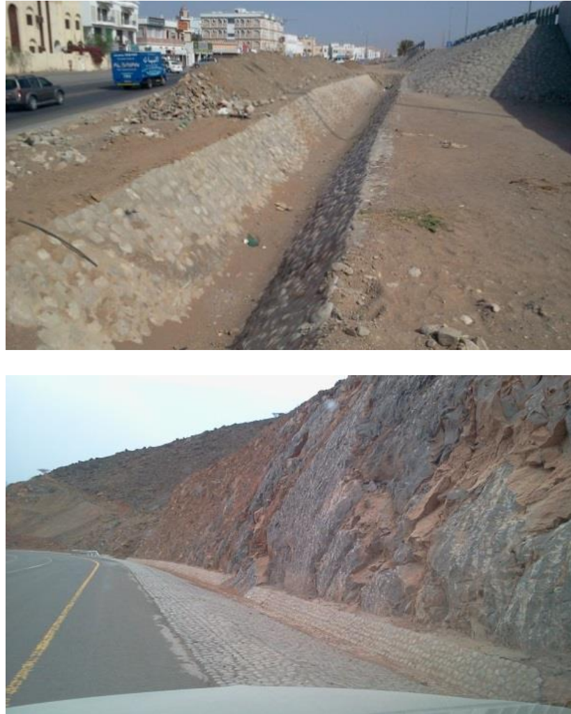
Figure 7.4: Drainage channel parallel to the main streets to drain the rainwater Source: Author's own
