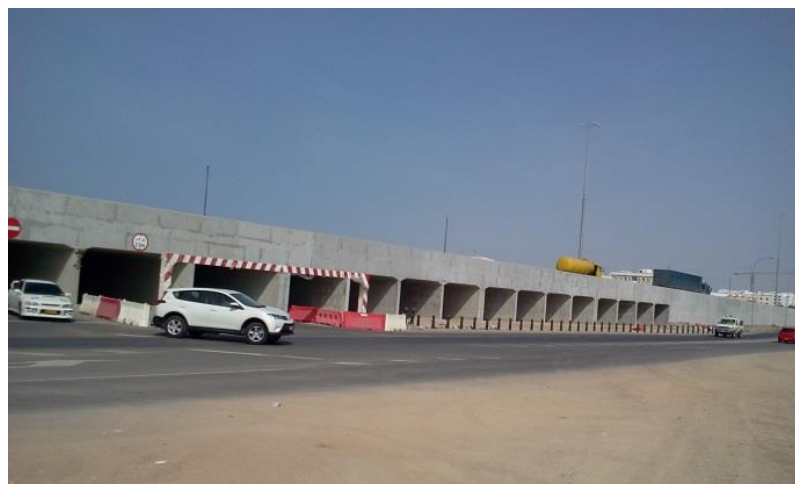
Figure 8.15: The huge culverts oriented towards houses and commercial buildings and used as tunnels for cars
