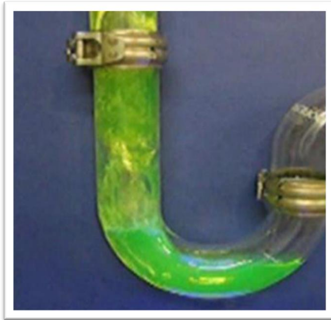
Figure 7. 2, Observation of the displacement of water in the appliance trap in the Heriot watt University drainage laboratory.
