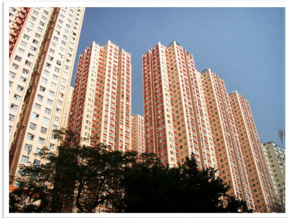
Figure 2. 9, Amoy Gardens housing complex, Hong Kong. Source, SKK (HK), (2015).
