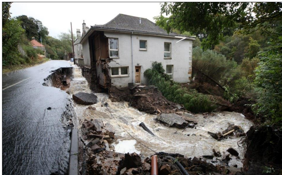
(a) Building fabric damaged in Fife floods in 2012 (© Gall, 2012 – Daily Record website)
