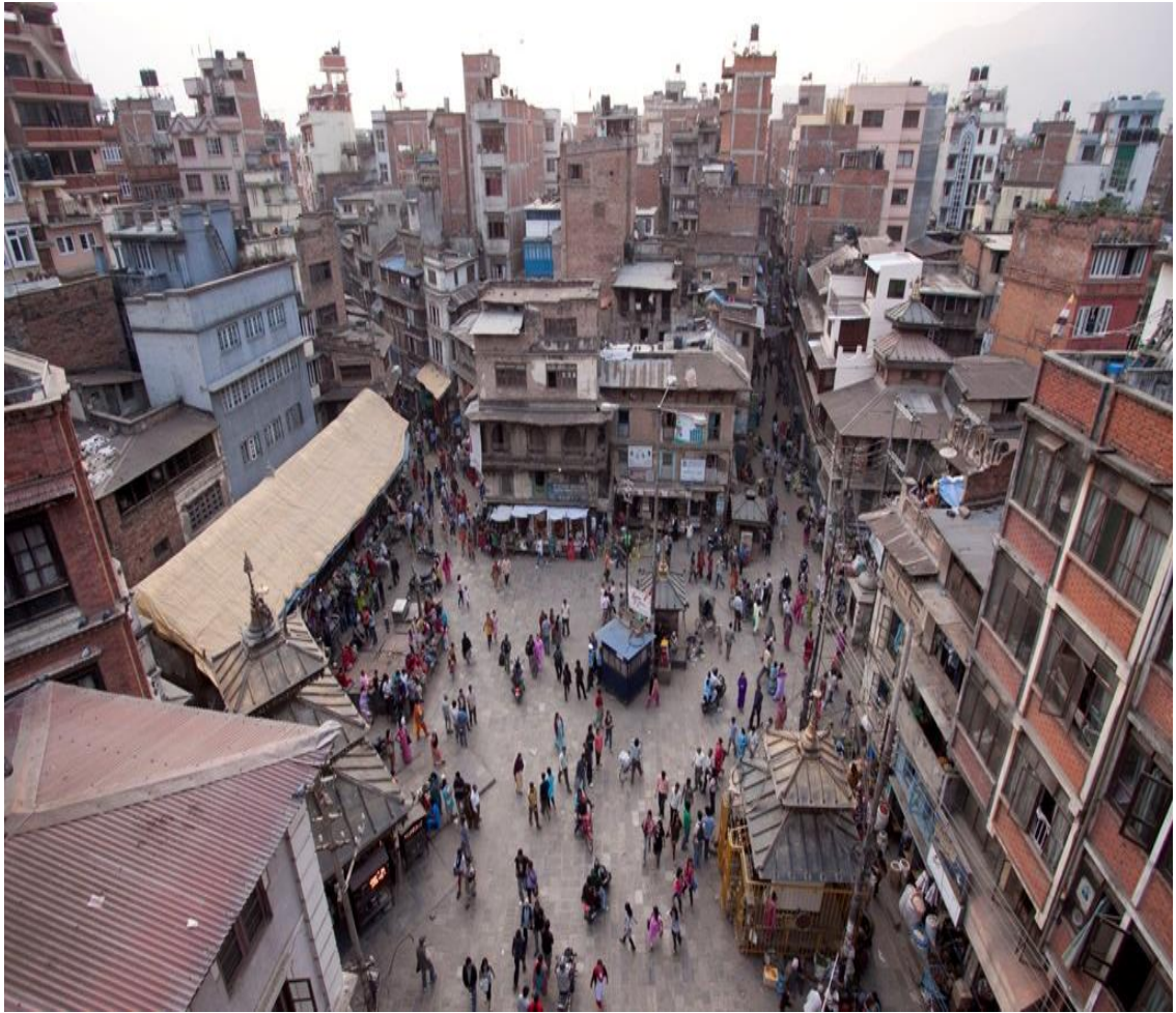
Figure 6.17: View of Ason looking west
