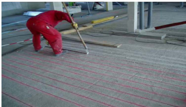
Figure 2.14 Near Surface Mounting Reinforcement, NSMR, in Stuttgart, Germany (Motavalli & Czaderski, 2007)
