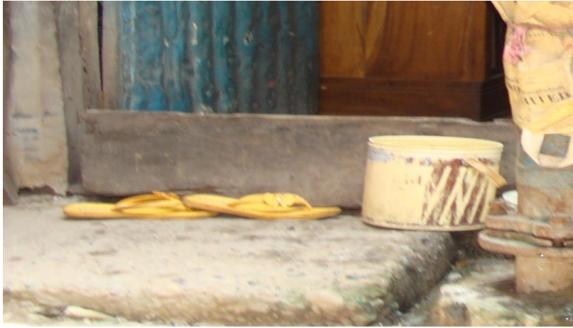
(h) Barrier at door. Source: Author's field survey, 2012
