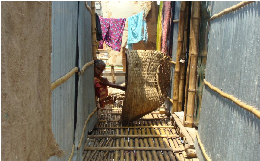
(e) Bamboo made floors of the stilt house. Source: Author's field survey, 2012
