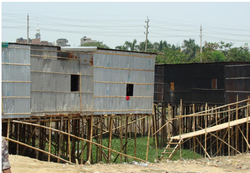
Figure 5.10: Hanging Shelters in Kamrangirchar
