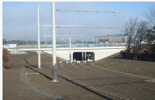
A8 Roadway Tunnel
