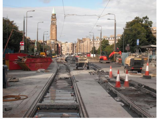
Concrete bed stripped off
