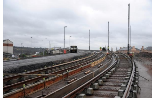
Tracks over the Carrick Knowe Bridge
