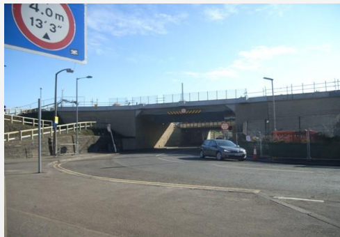
Russell Road Bridge
