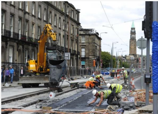
Concrete bed re-laid in progress
