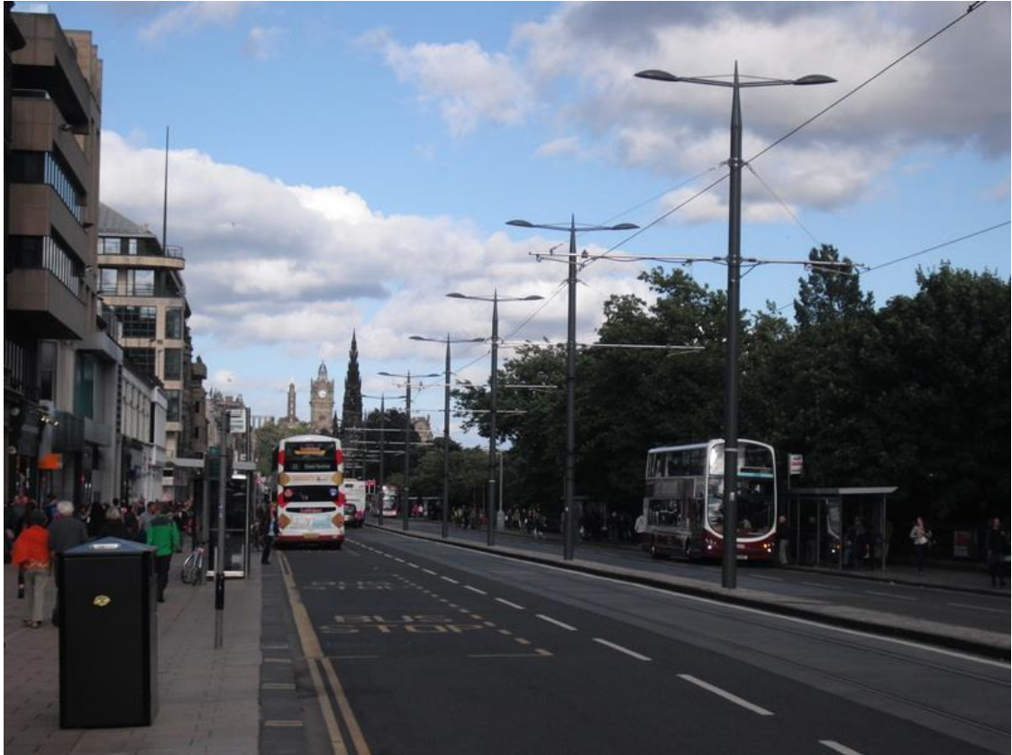
Exhibit 4: Overhead Electric wire installation on the Princes Street
