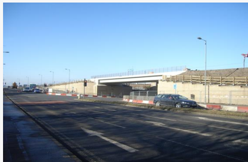
South Gyle Access Bridge
