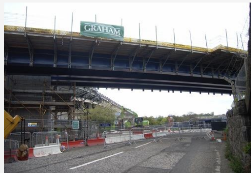
Murray field Viaduct under construction
