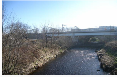
Water of Leith Bridge situated between Balgreen road and Murray field tram stops
