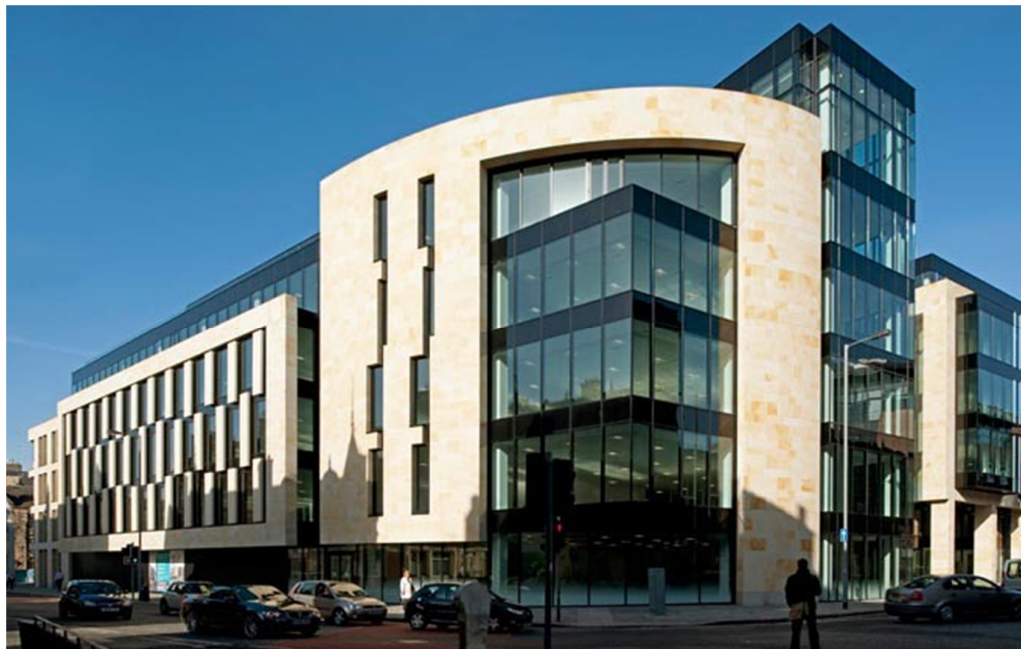
Figure 29 - Case study building B view from southeast (Google, 2010)
