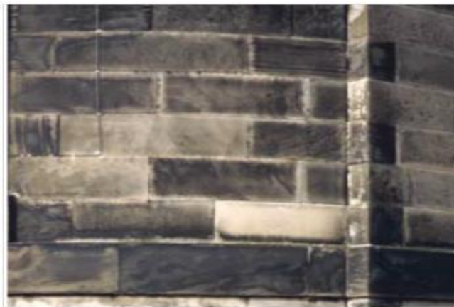
Figure 2.6: Typical example of ashlar masonry with ashlar mortar joints Source: Historic Scotland, 2007a.
