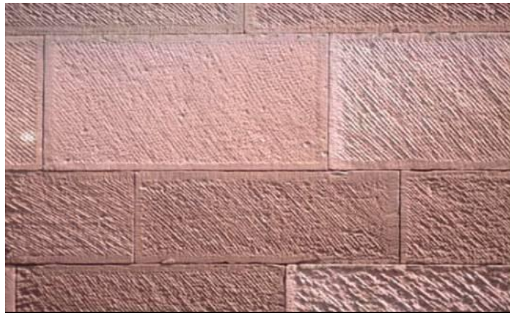
Figure 2.8: Typical example of stone tooling effects
