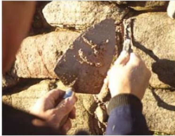
Figure 2.14: Repointing process rubble stonework
