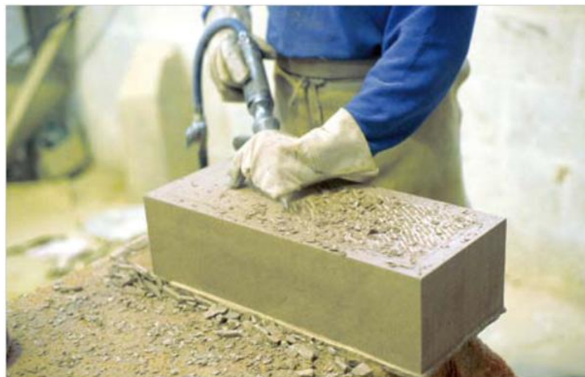
Figure 2.7: Tooling of ashlar masonry
