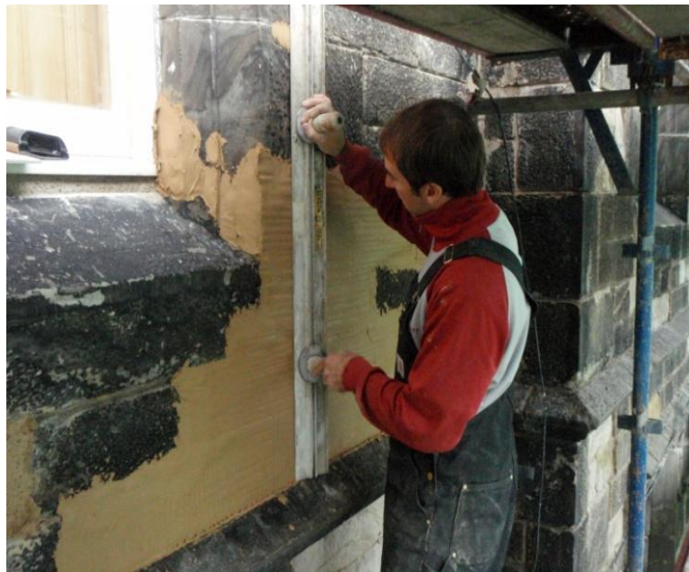
Figure 2.19: Execution of plastic repair to ashlar façade, Edinburgh.
