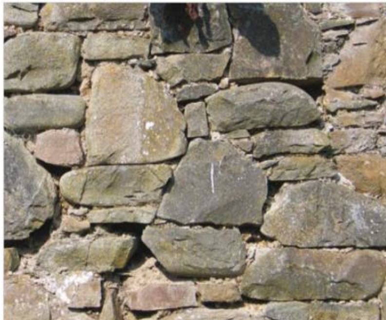
Figure 2.5: Typical example of rubble masonry with lime mortar joints Source: Historic Scotland, 2007d.
