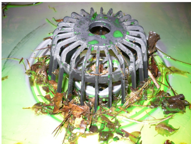
Figure 5.4(b) Outlet B, after loose detritus test.
