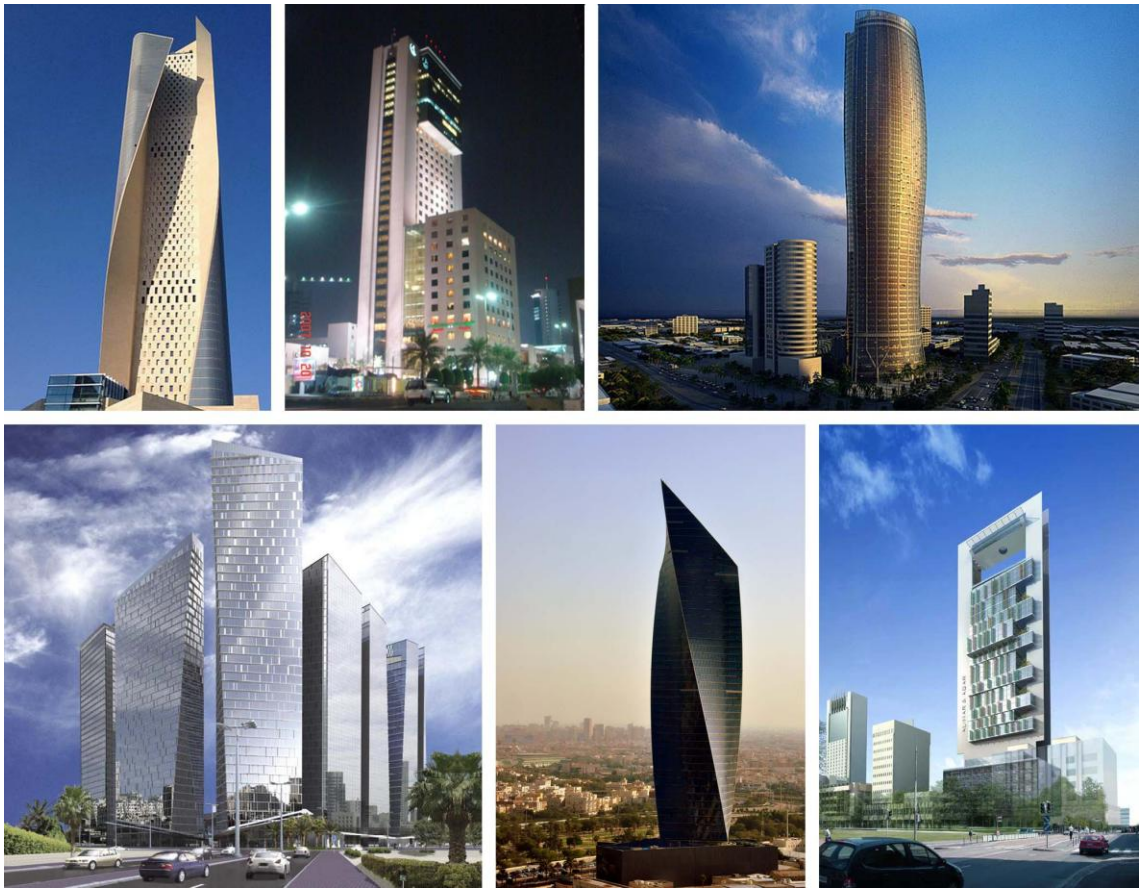
Figure 7. 4 Office Towers in Kuwait City. (Sources: businessinsider.com , panoramio.com , p0ech.com , fried-junk.com , isul6ana.com & e-architect.co.uk )
