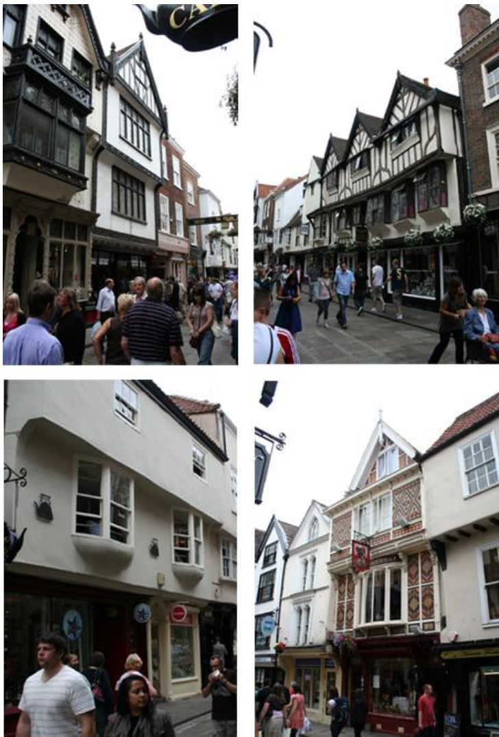
Figure 5. 20 High-quality Historic Architecture on Stonegate (Author)
