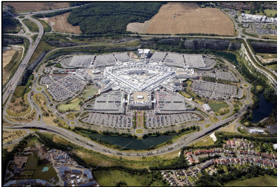
Figure 2.12 Bluewater Shopping Centre (source: http://www.heritage-explorer.co.uk )
