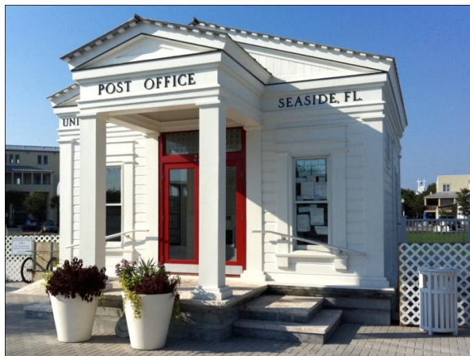
Figure 3.13 Post Office Building at Seaside, Florida (Source: http://mattnt.com )
