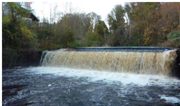
(c) Large weir (Dean Village)
