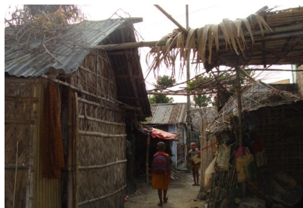
Railway Slum: In Railway slum, the use of CI sheet on the roof is a common picture and use of bamboo and straw in the wall material also indicates the use of local materials to reduce the cost of construction.
