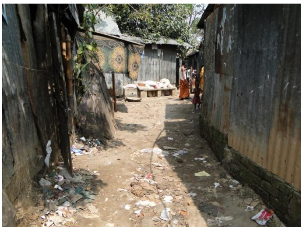
Karail Slum: In Karail, the access road is footpath only. This access road is not paved and becomes muddy in the rainy season.
