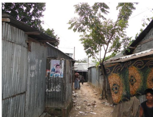
Karail Slum: As discussed in chapter six, most of the dwellings in Karail are made of CI Sheets.
