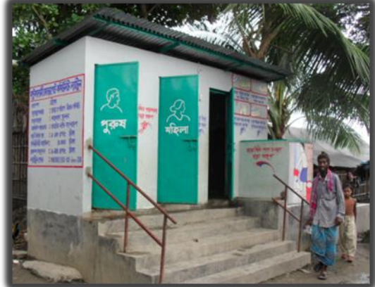
Railway Slum: In Railway slum, NGO provided communal latrine is the dominant type of sanitation which has different provisions for men and women.
