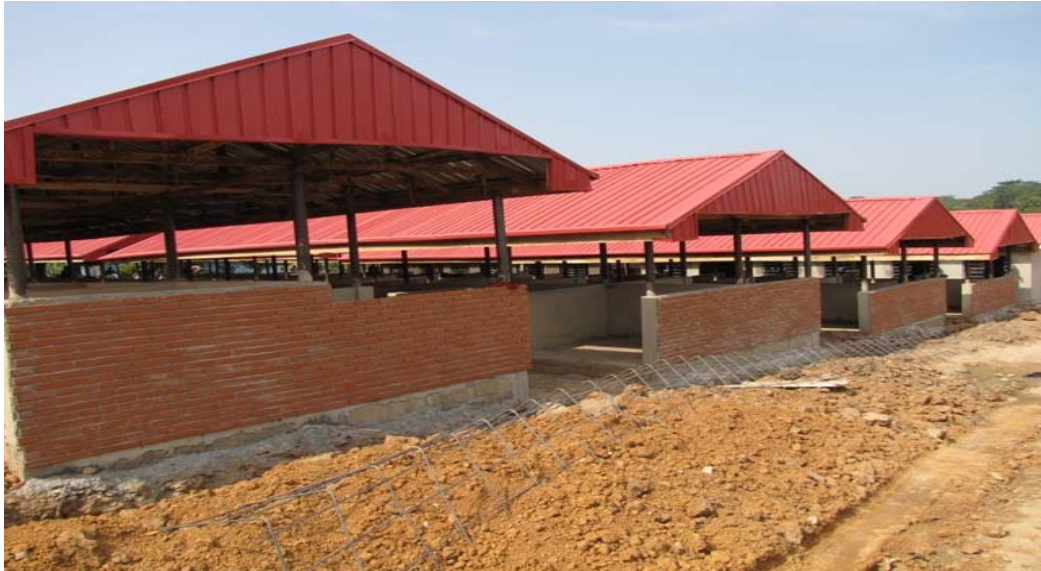
Figure 8.10: Neighbourhood market in Isinkan, Akure
