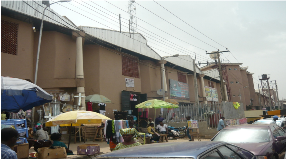
Figure 8.3: Front view of Erekesan Market in Akure.
