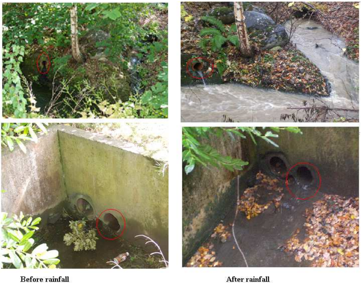
Figure 3.2: Additional flow to the Murray Burn stream through Campus drainage systems during rainfall events.
