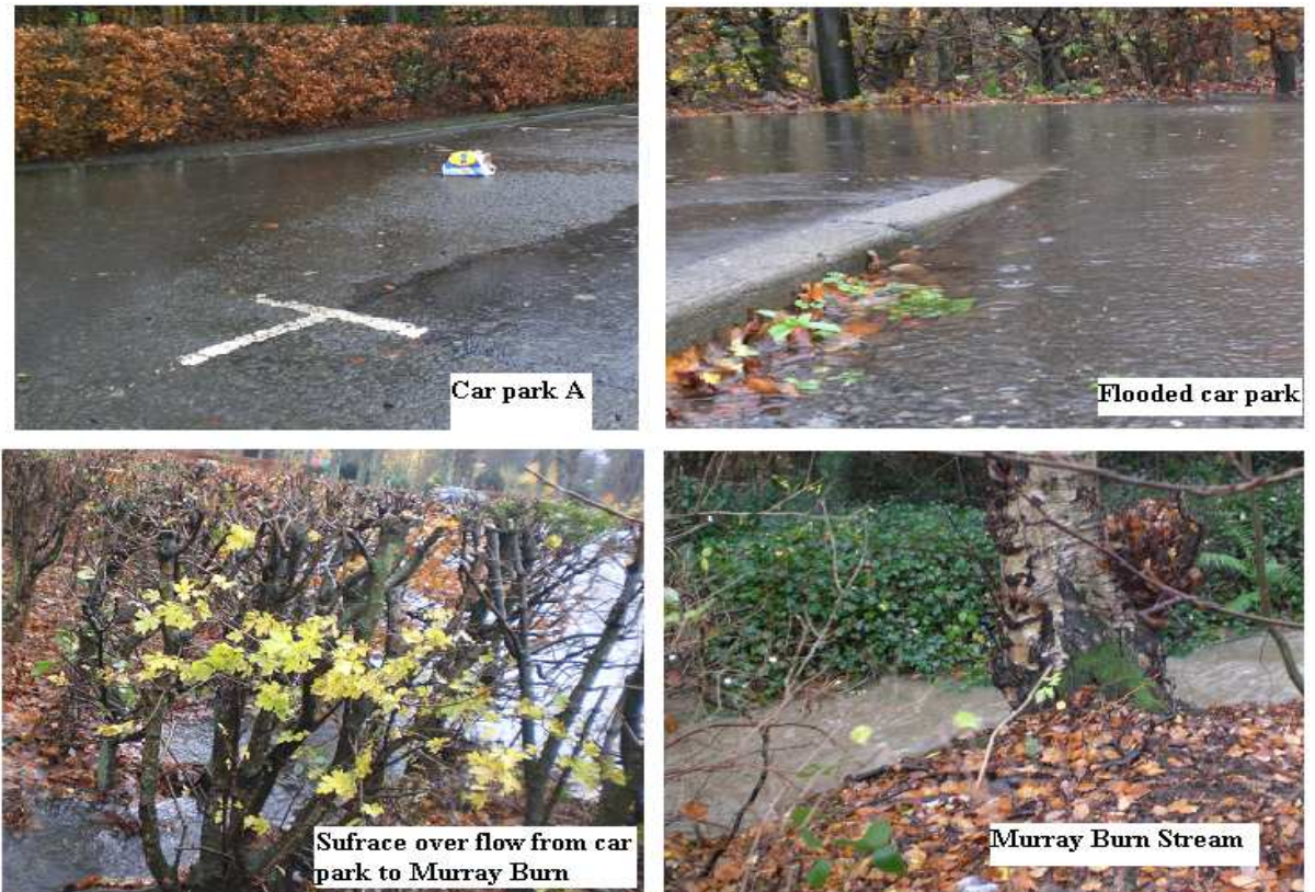
Figure 3.3: Surface overflow from Car Park A to Murray Burn during rainfall events.
