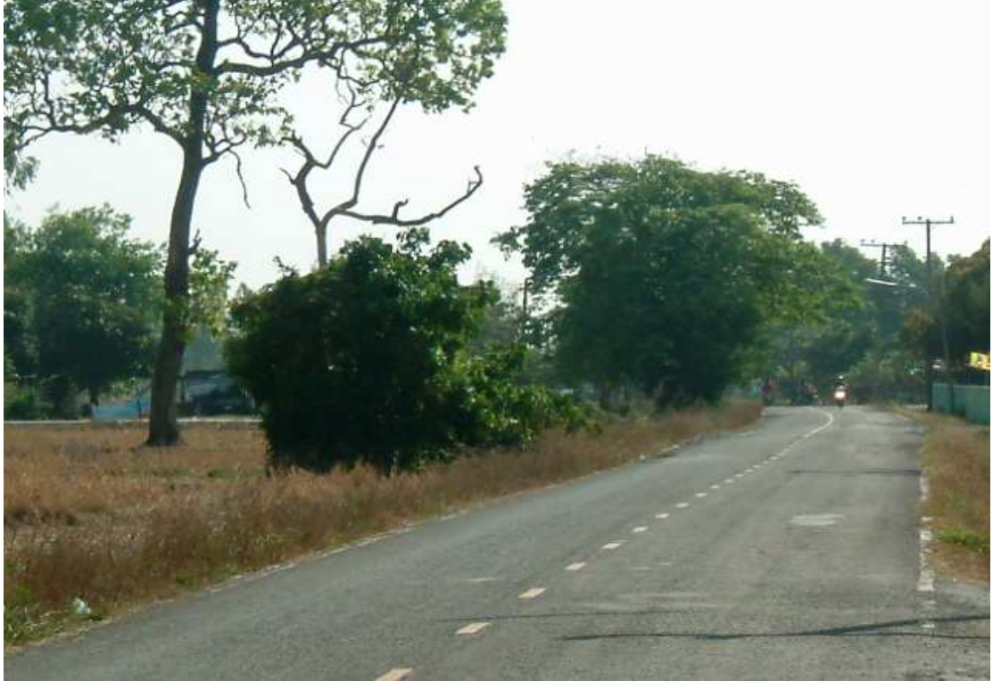
Figure 9.12: A two-lane concrete road in the village; (source: author's survey)
