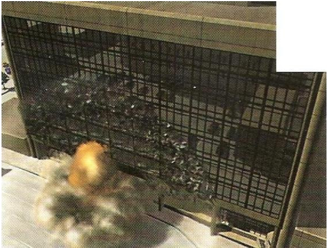
Figure 3.3b: Computerized simulation of blast wave as it shattered the glazed façade of the Alfred P. Murrah Federal Building, after Wearne 1999
