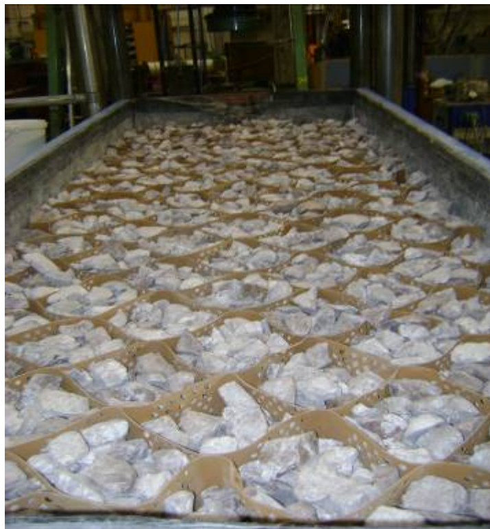
Figure 5.18. Geocell ballast layer prior to compaction and placement of top layer of ballast
