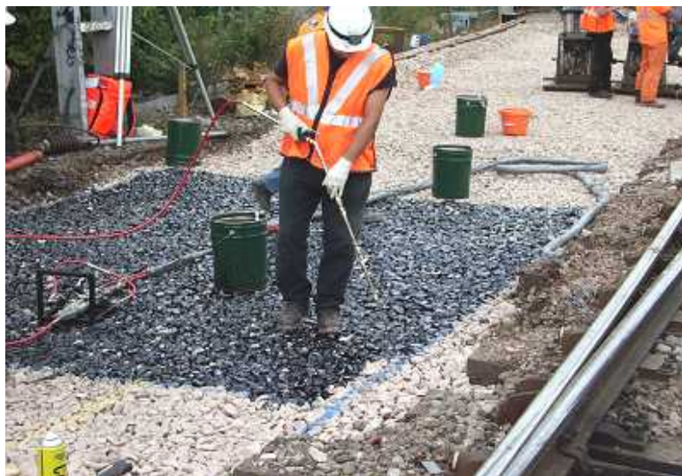
Figure 2.8. Typical XiTRACK application on site (XiTRACK Ltd, 2010)
