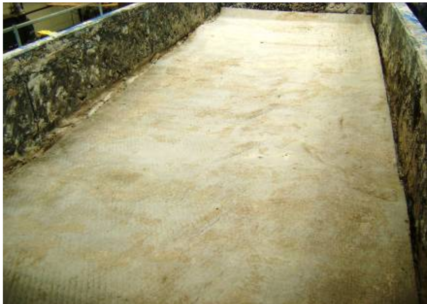
Figure 5.34. Full geocomposite layer on formation
