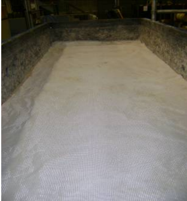
Figure 5.22. Reinforced geocomposite placed in GRAFT
