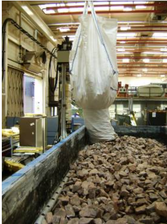
Figure 3.23. Ballast placement from one tonne bag
