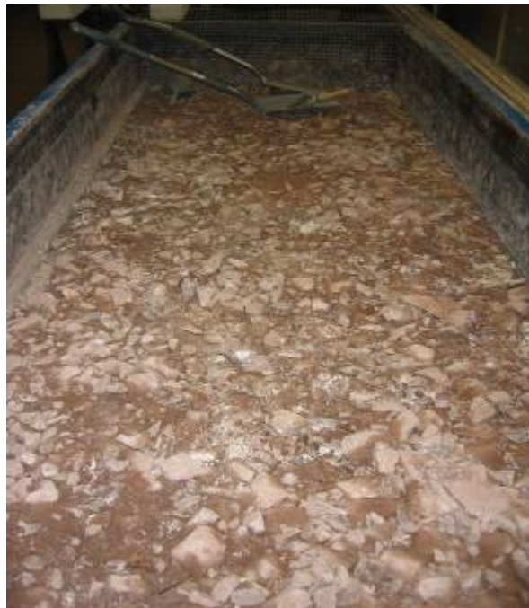
Figure 3.27. Penetration of formation layer with ballast particles after flooding test
