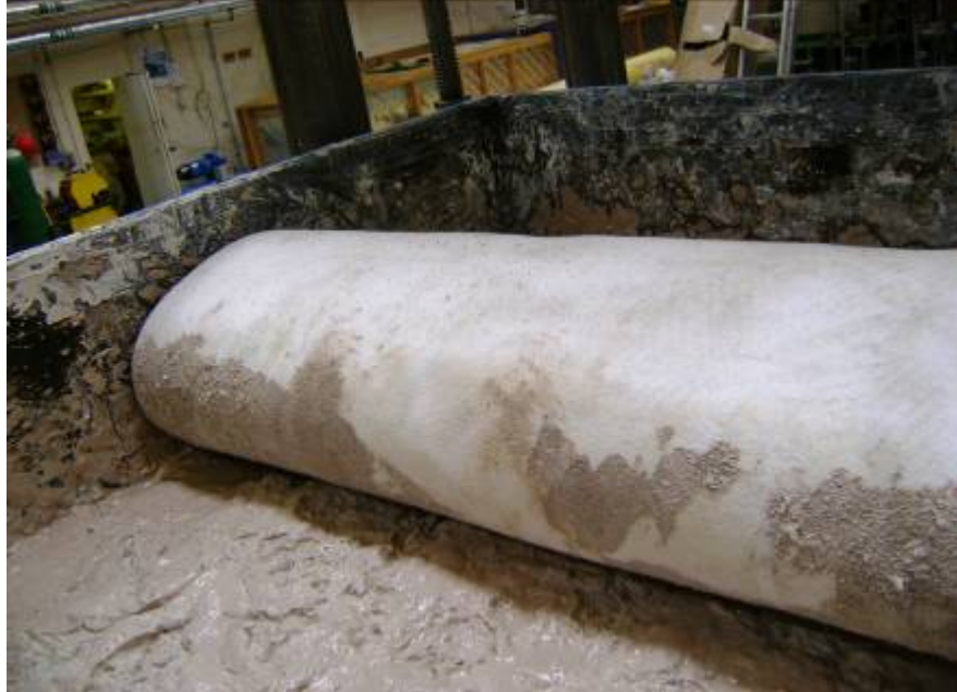
Figure 5.33. Placement of geocomposite on slurred formation
