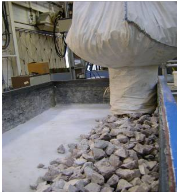
Figure 5.23. Placement of ballast on top of reinforced geocomposite
