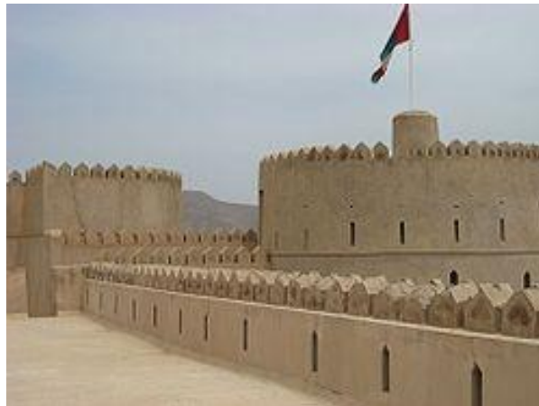
Figure 7:4 The Al-Rustaq Fort (The Ministry of Information, 2008)
