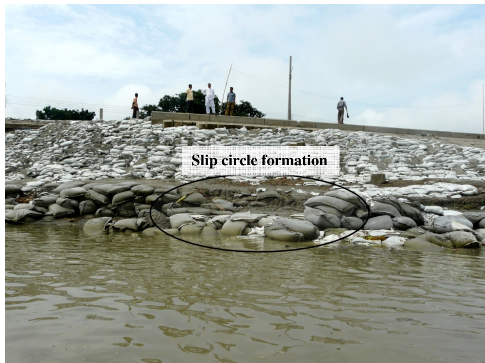
(b 1) Bag displacement due to combined effect of retarded scour and drawdown
