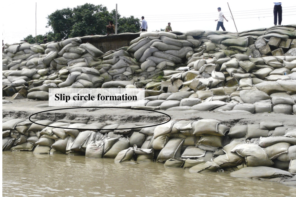
(a 1) Displacement due to rapid drawdown
