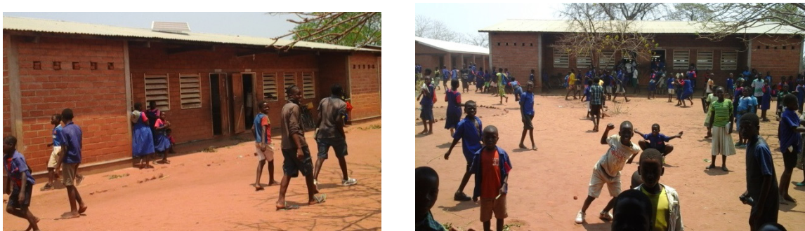
Photos: Solar PV installed at school blocks at Nkasi Primary School
