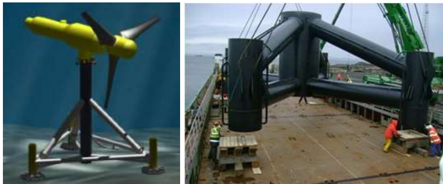
Figure 14: Pin pile foundation configurations ( left ) Alstom/TGL 1MW turbine (image source: [38]) and ( right ) Lifting of the MCT SeaGen quadrapod foundation
