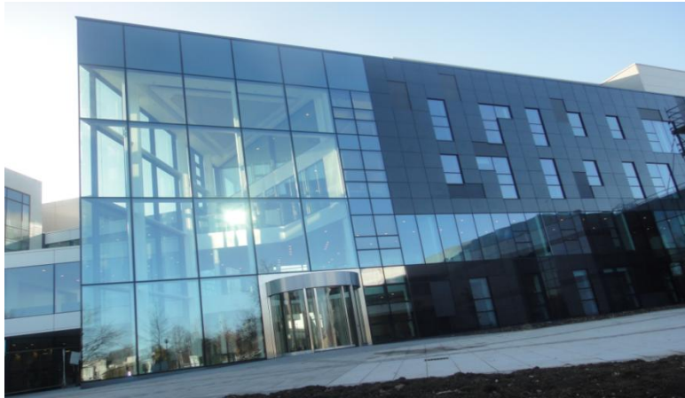
Fig. 1 Completed Charles Institute Building
