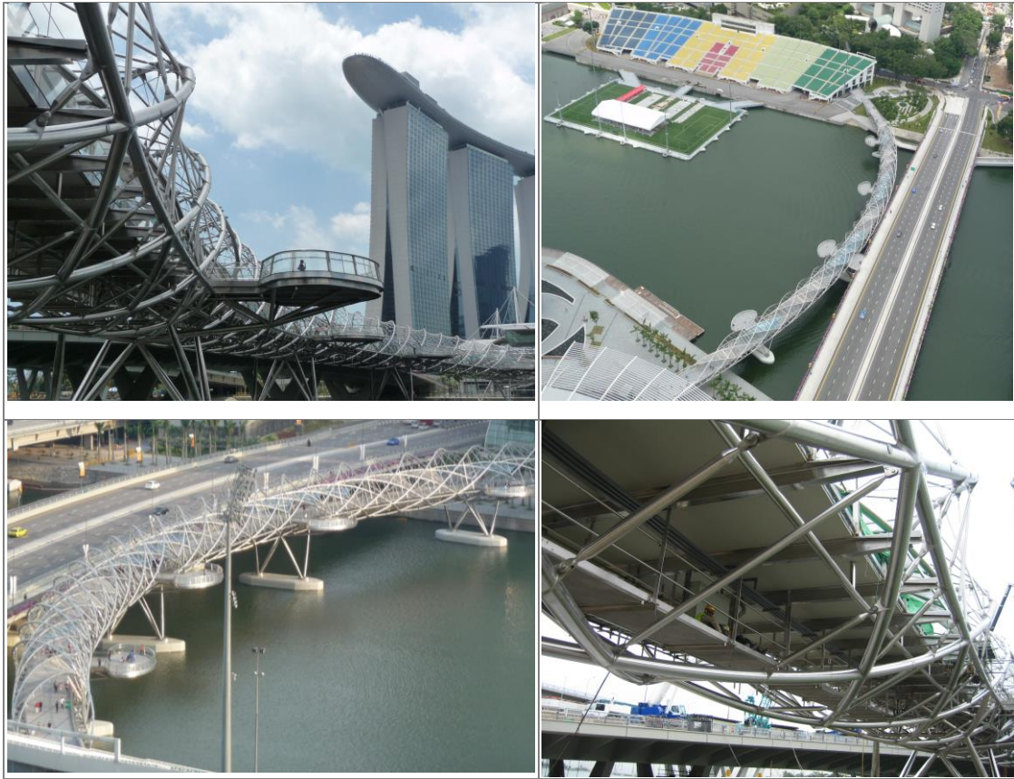
Figure 1: Helix Bridge. Clockwise from top left. View from Esplanade showing pod, Marina Bay Sands Hotel and Skypark; View from Skypark showing Marina Bay and stadium for National Day celebrations; Detail of helical framing system and walkway support; View from (distant) high-rise hotel showing pods, piers and columns.
