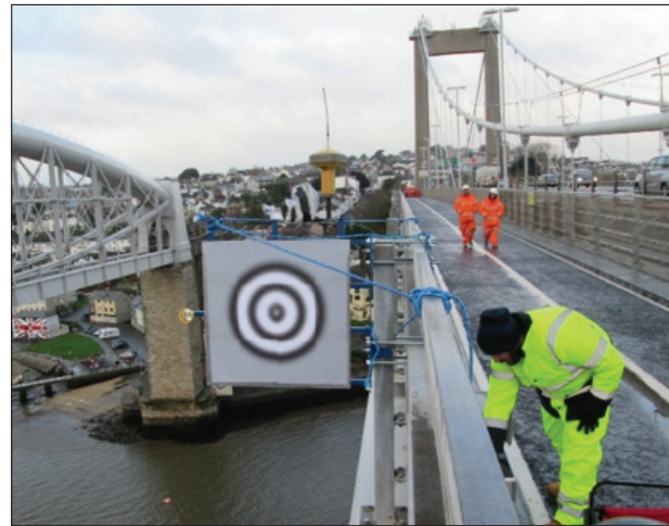
Figure 7: Mounting configuration of target frame at mid-span
