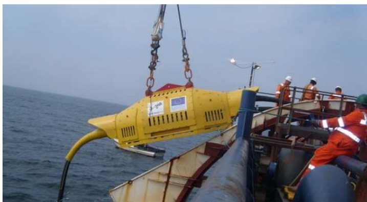
Figure 7 : Wave Hub connector deployment
