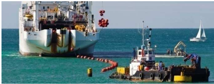
Figure 6: SEMREV Testing site Power cable laying (credit Orange Marine)
