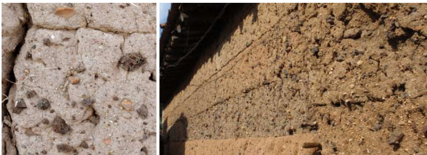
Fig. 7 Past metal-working within settlements is often evidenced by slag and crucible fragments embedded in house and compound walls. While this is recorded as secondary deposition it is rare that the mud used in building construction travels far from its point of origin.
