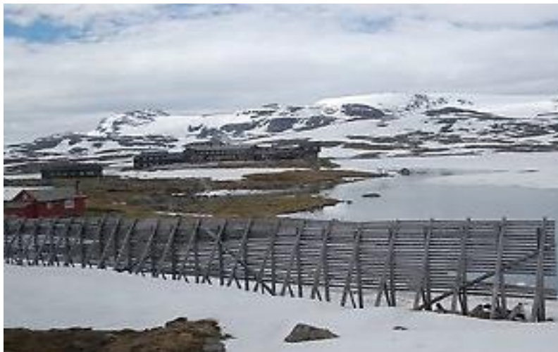
Figure 1-2: Snow fences to protect the driveway in Norway
