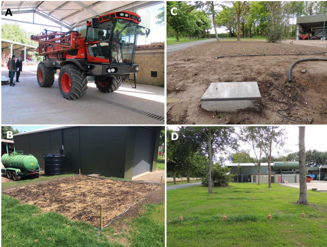
Figure 2: Images of the biobed facility installed at Manor Farm, Salle. (A) Pesticide sprayer inside the machinery wash-down unit during construction; (B) biobed operational area (7 m x 7 m) with the completed enclosed wash-down unit in the background; (C) biobed output sump and trickle irrigation system during construction; (D) drainage field trickle irrigation area, with porous pot outlets located underneath terracotta pots.
