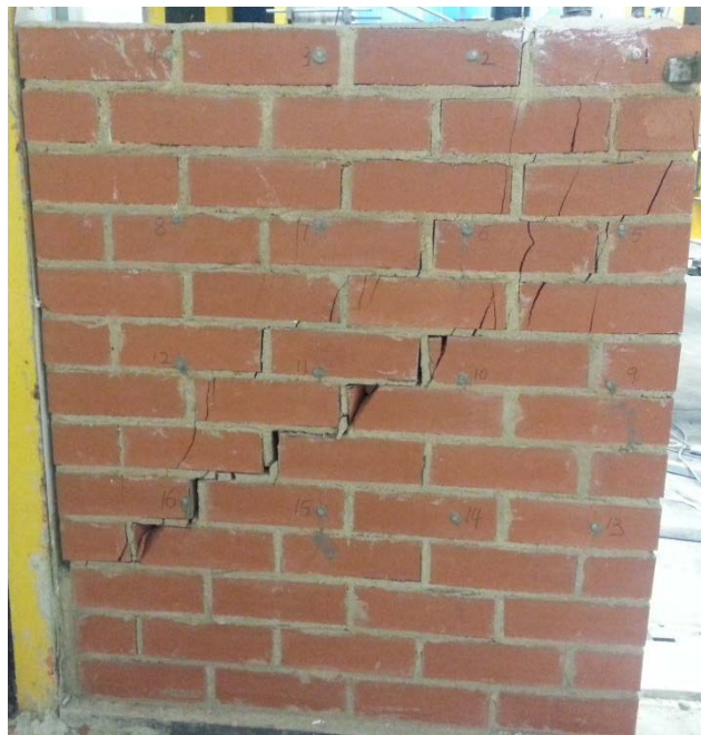
Figure 7.22 Experimental deformation of collar jointed wall W7 on the front side
