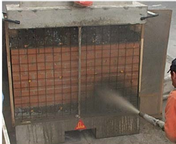
Figure 2.12 Application of shotcrete to URM wall (EIGawady et al. 2006)
