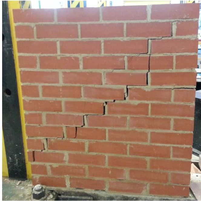
Figure 4.8 Failure pattern of double-leaf wall W5 on the unloaded leaf
