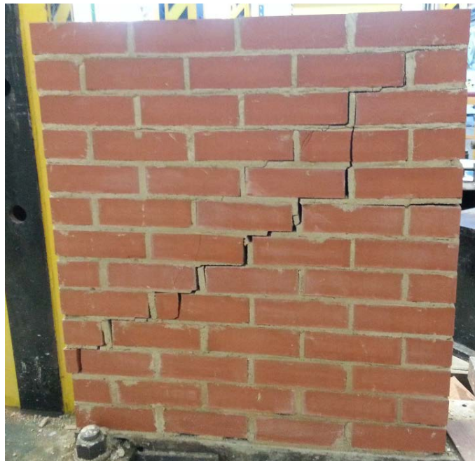
Figure 7.13 Experimental deformation of collar jointed wall W4 on the back side
