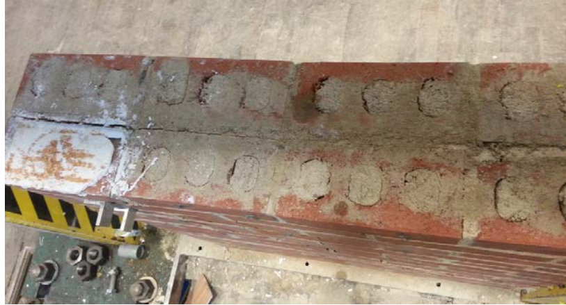
Figure 4.12 Failure pattern of the collar joint on top side of W5
