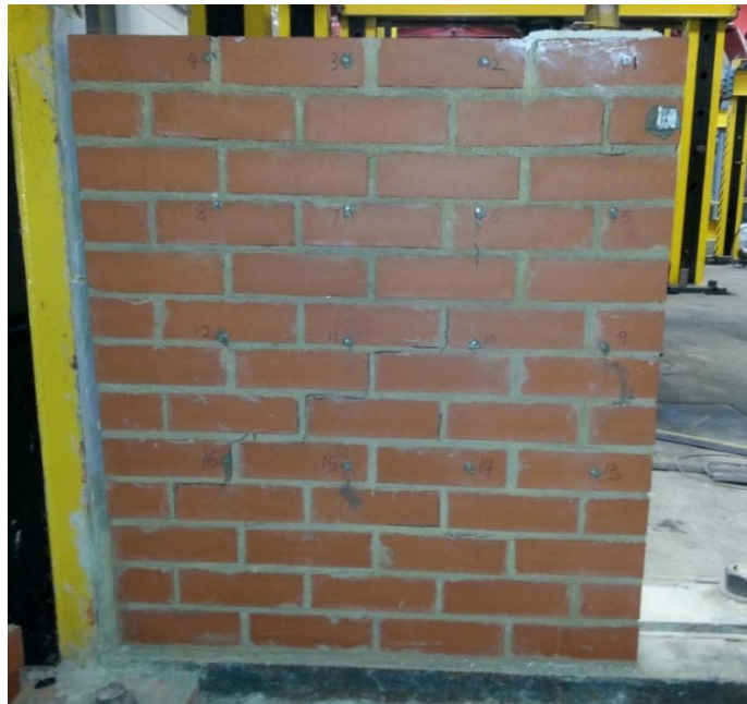
Figure 4.4 Failure pattern of single-leaf Wall 6
