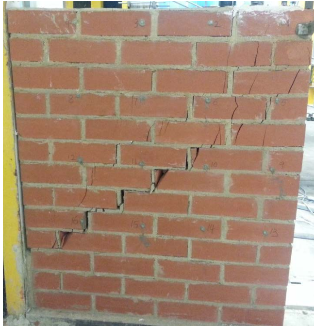
Figure 4.9 Failure pattern of double-leaf wall W7 on the front side
