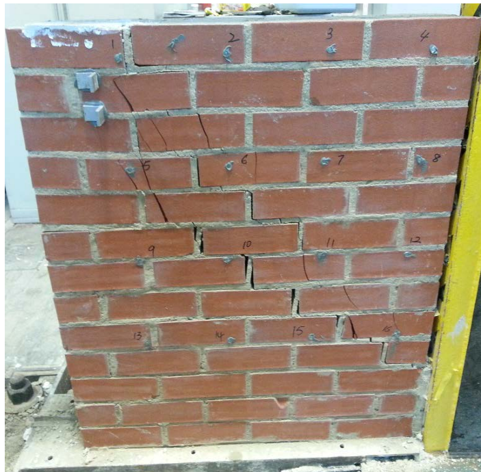
Figure 7.11 Experimental deformation of collar jointed wall W4 on the front side
