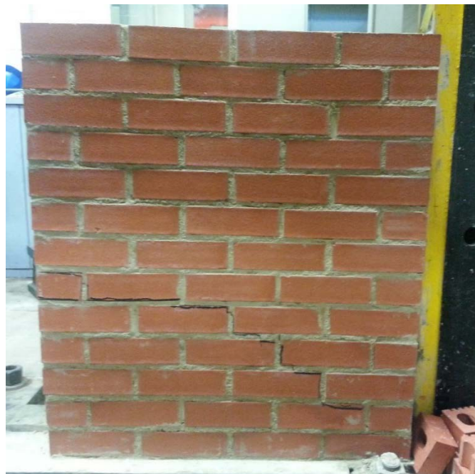
Figure 7.24 Experimental deformation of collar jointed wall W7 on the back side
