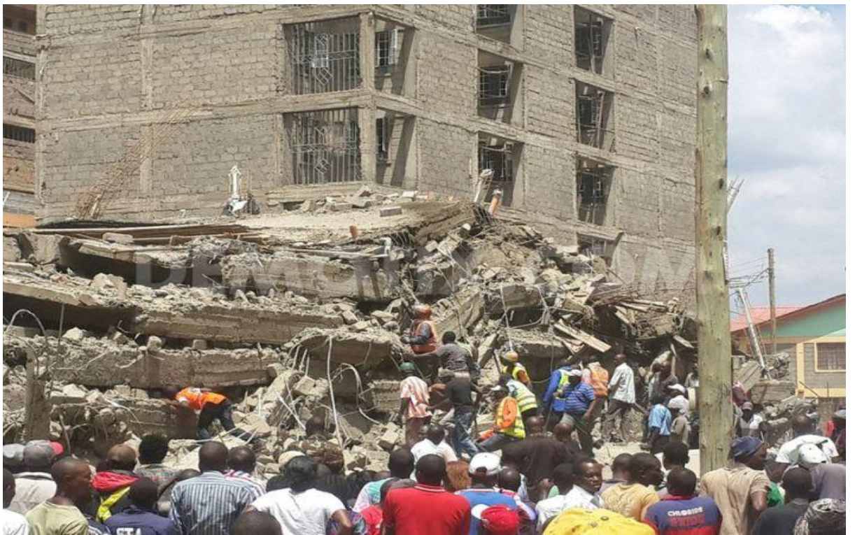
Figure 5: Collapsing buildings in Nairobi (the-star.co.ke, 2015)
