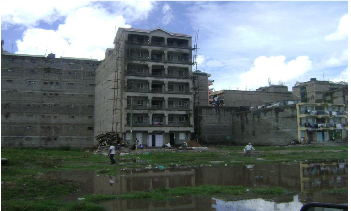
Figure 7: Drainage problems in Eastlands (Author, 2014)
