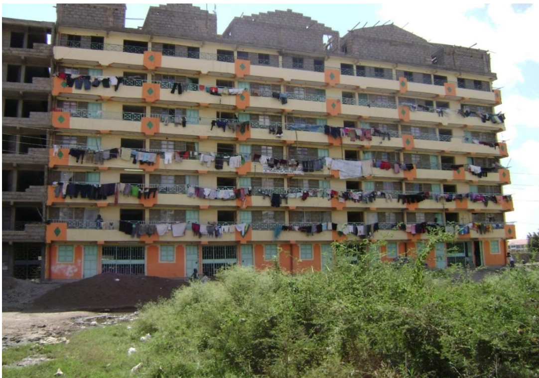
Figure 22: An incremental building in Eastlands; evidently occupied but additional floors being built (Author, 2014)
