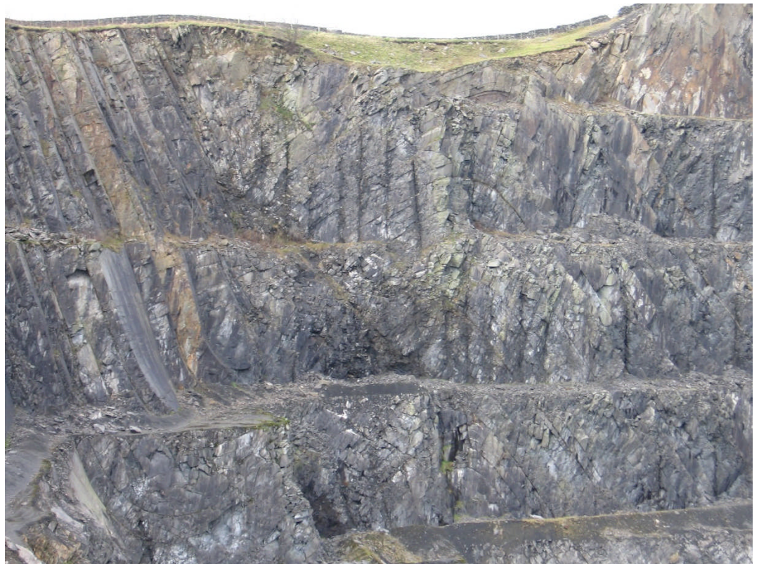
Figure 3.3 West exposure of DRQ showing a fold structure and incipient discontinuities including inclined beds and joints.
