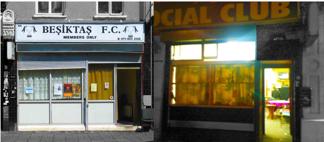
A combination of curtains and roller shutters provide privacy; a built-in shelf and curtains provide screening and also a display area.
