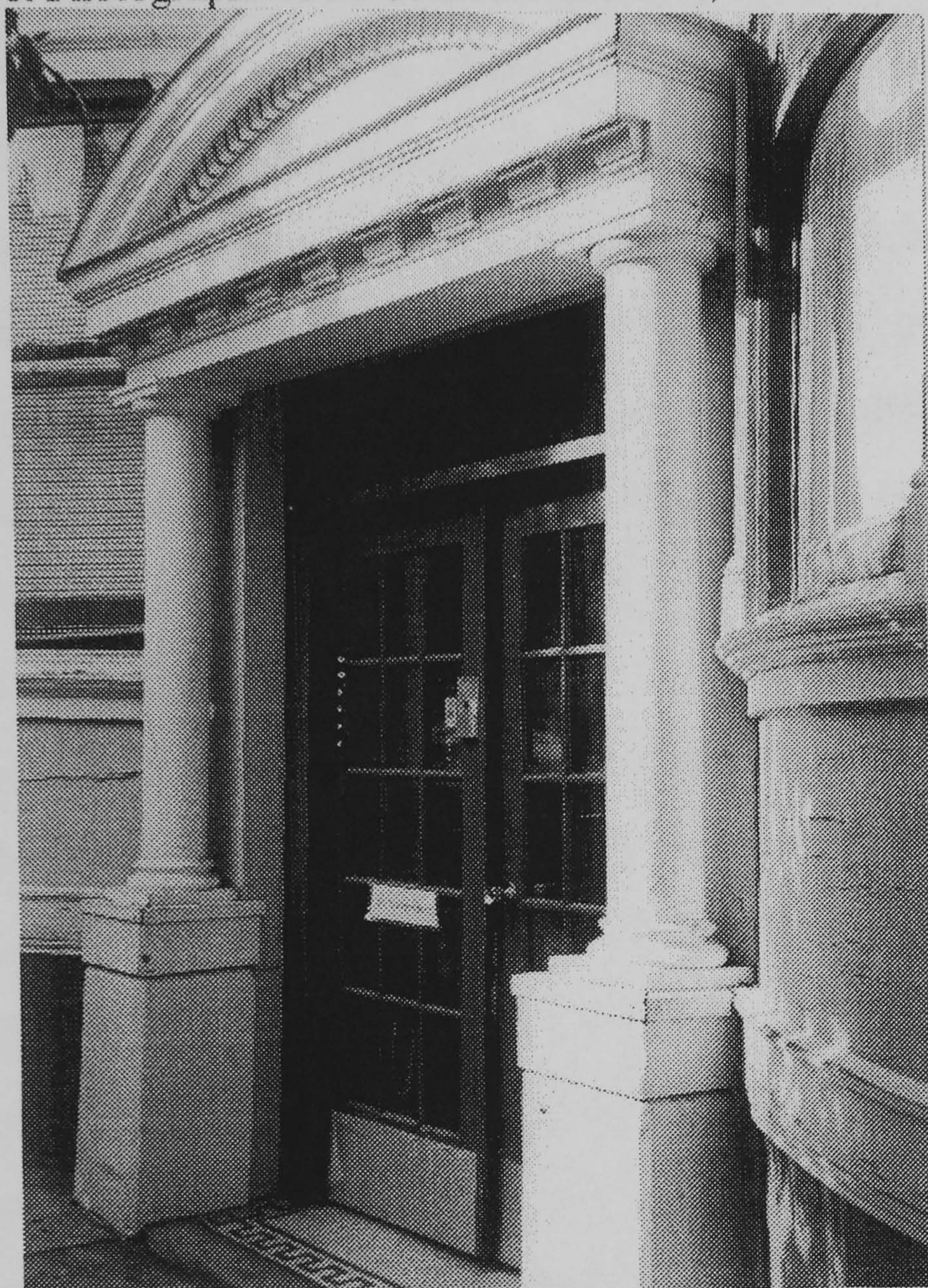
Figure 46. Photographs of 20 Cumberland Street, San Francisco.
