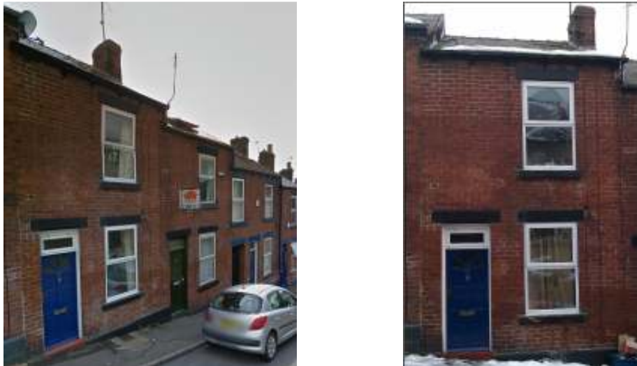
Figure 3.3: Victorian terrace house used in this work.
