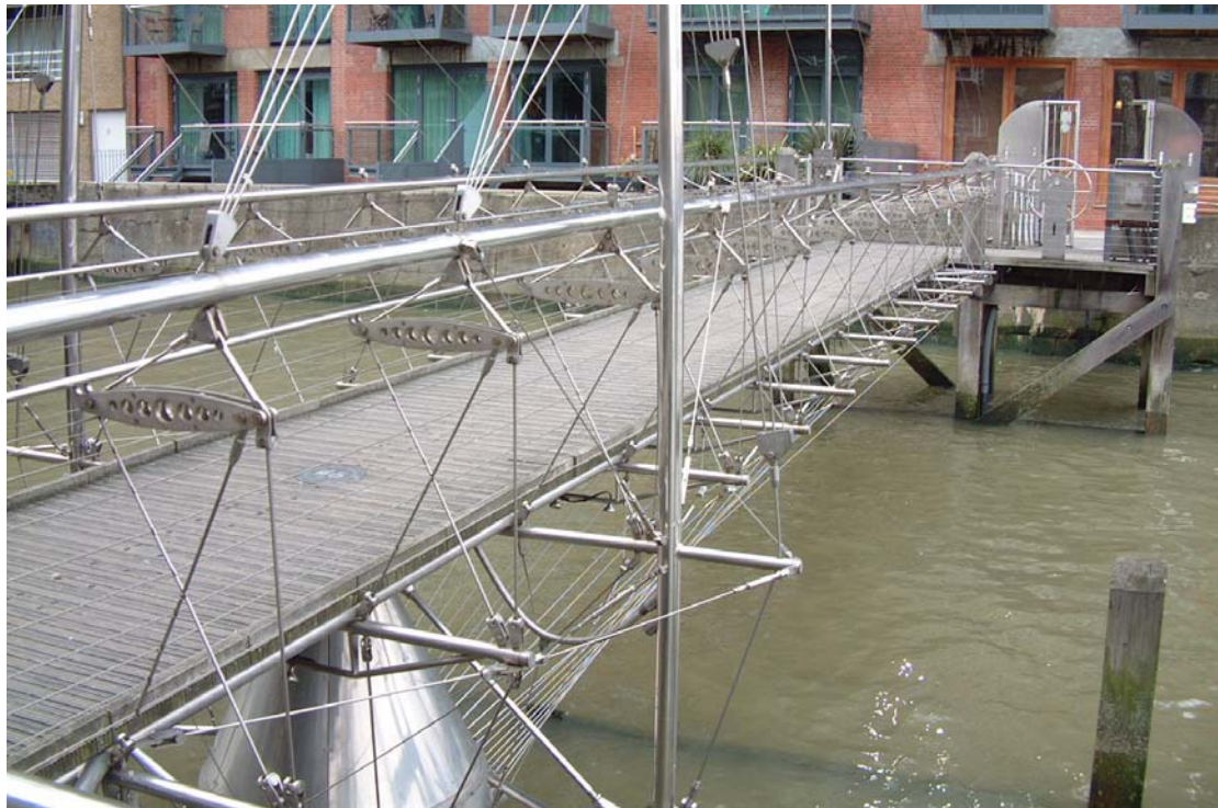
Figure 7 Stainless steel bridge, St. Saviours Dock, Shad Thames, London
