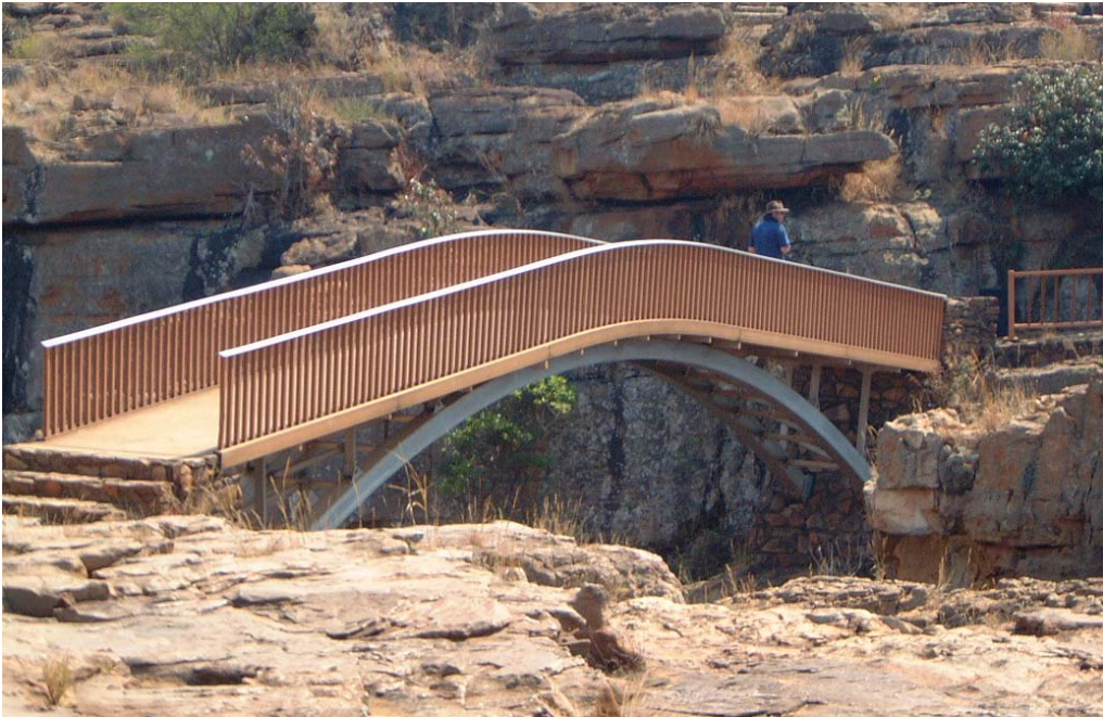
Figure 6 Aluminium alloy bridge, Bourke's Luck, South Africa
