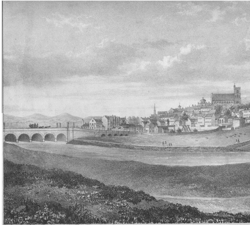
Fig. 4. 1832 engraving of the Eden Bridge completed in 1815, showing the main five arch span over the Eden and the second bridge over the dry branch of the Eden. From Cumbria Image Bank (Cumbria County Council, 2014).
