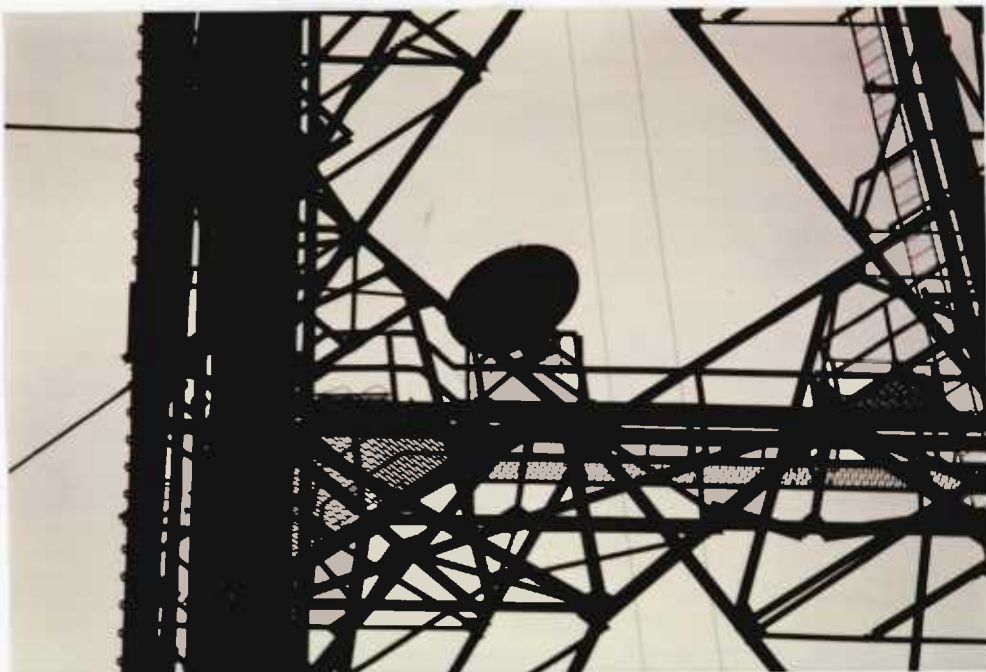
Fig. 6.4b: Transmitter fixed at 90 meter level!
