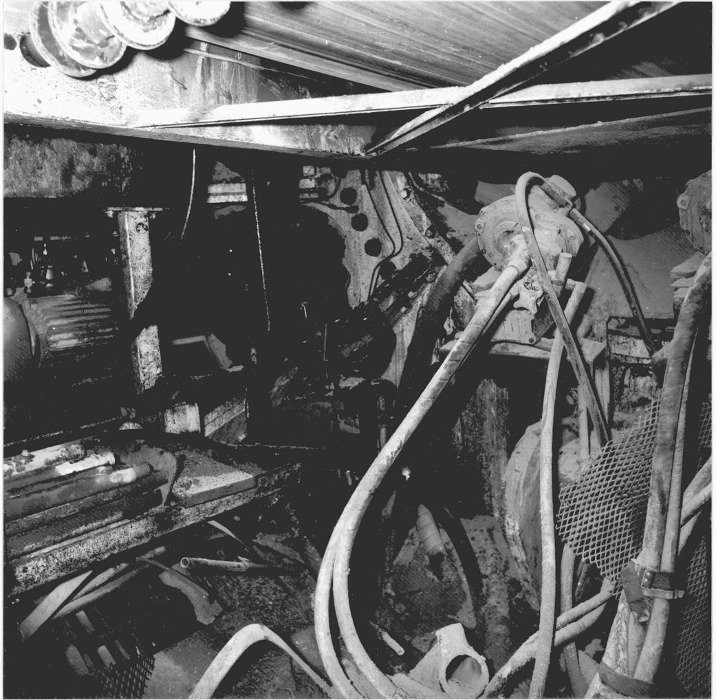
PLATE 13 Working space for probing ahead on the Channel Tunnel machine
