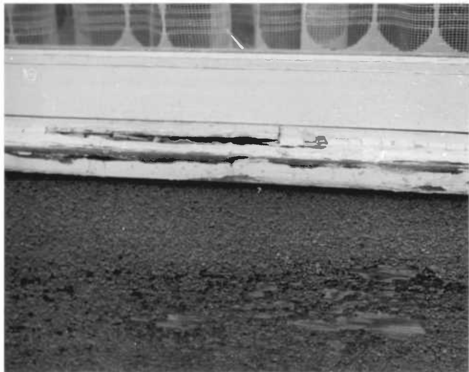
Fig 2.13 Larkhill; decay of a sill associated with the centrally positioned butt joint
