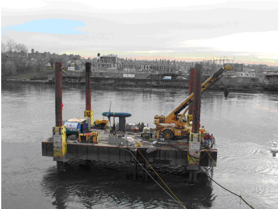
Figure 176. Jack-Up Barge for Installing Turbines and Transducers
