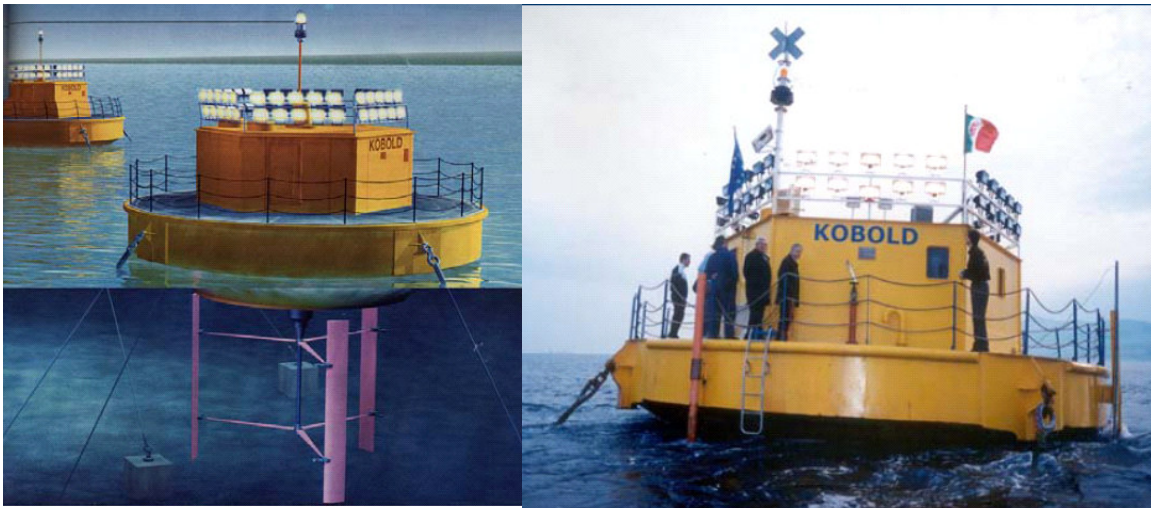
Figure 42: Darius-Type Tidal Turbine - the "Kobold"
