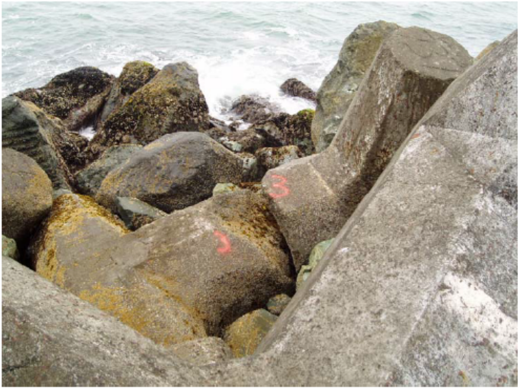
b. Example of middle-stem fracture.
