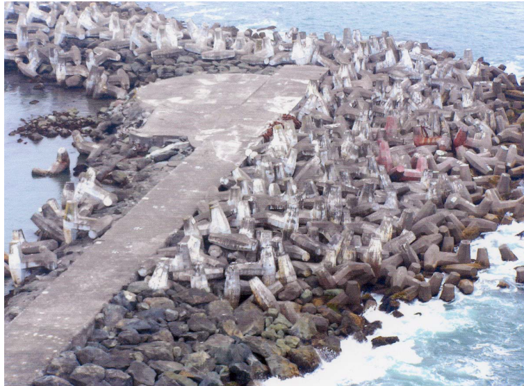
Figure 1: Crescent City breakwater covered by Dolosse units, California, USA (after Myrick and Melby, 2005). The weight of each Dolos unit is 38.1 t. The red units are instrumented with internal strain gages for monitoring purpose.
