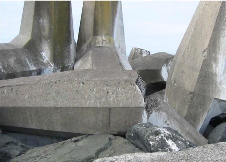
a. Example of fluke-stem fracture.
