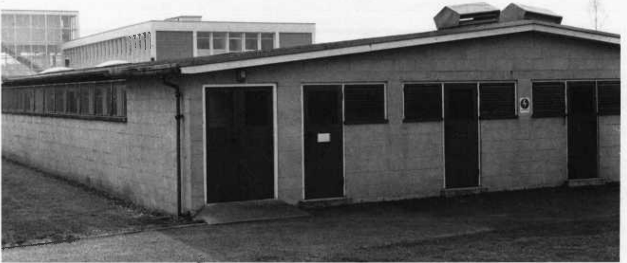
Fig.1 VIEW OF ISOLATION BUILDING FROM PLANT ROOM END
