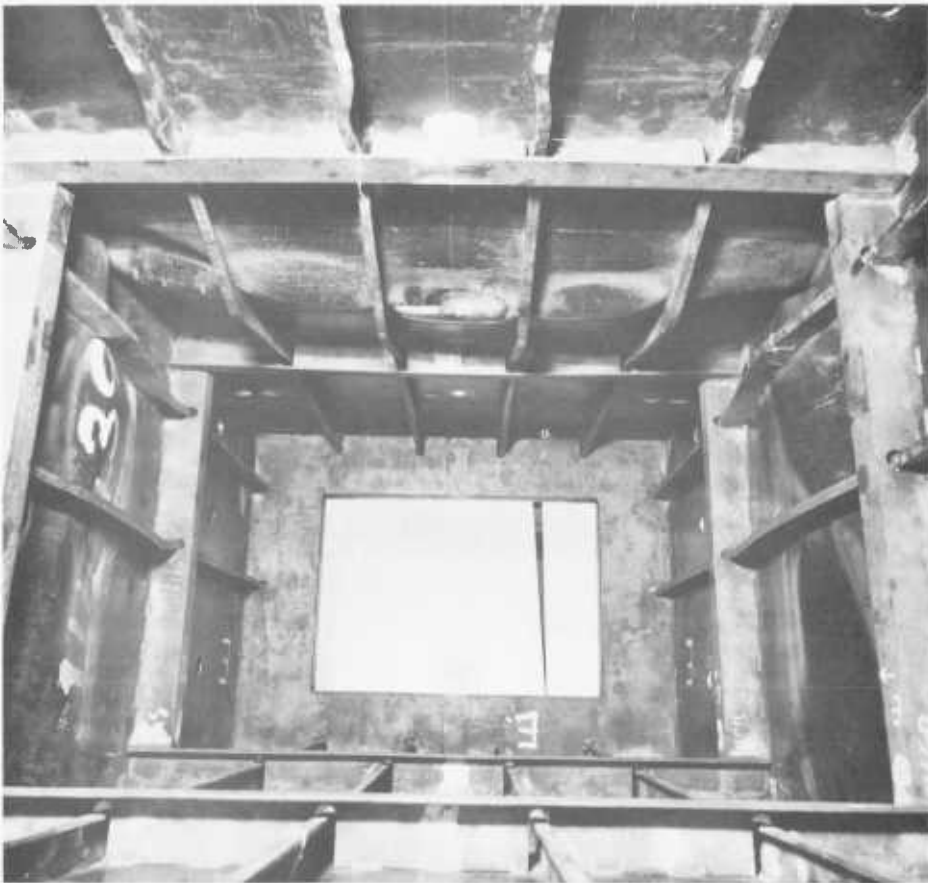
Fig. 2.33b. Model 2 - showing the interior of the model (from end C) after collapse. Note the lateral buckling of longitudinal stiffeners close to the transversals, in the bay adjacent to the critical one.
