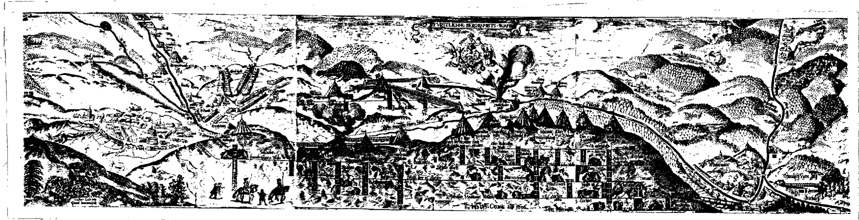
Panorama of the mines at Clausthal and Zellerfeld in the Upper Harz showing nineteen runs of field rods. Source: D. Lindemeier, engraving , 1606.
