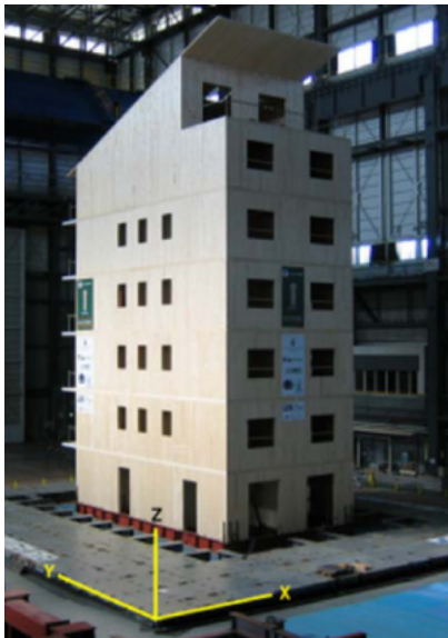
a) 7-storey CLT building (Ceccotti et al., 2013)
