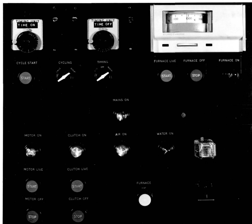
FIG.13. View of main control panel.
