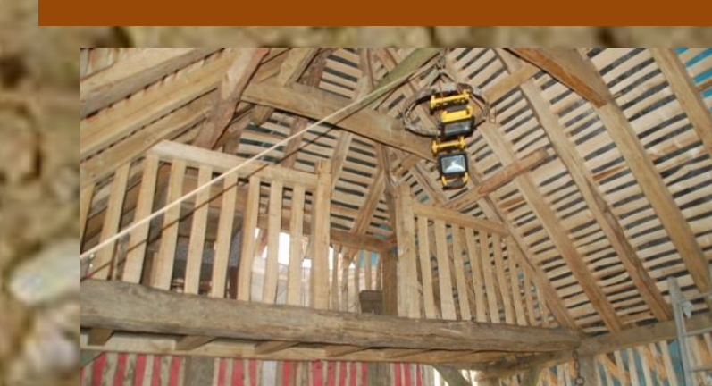
New mud & Stud cottage Near Skendleby
