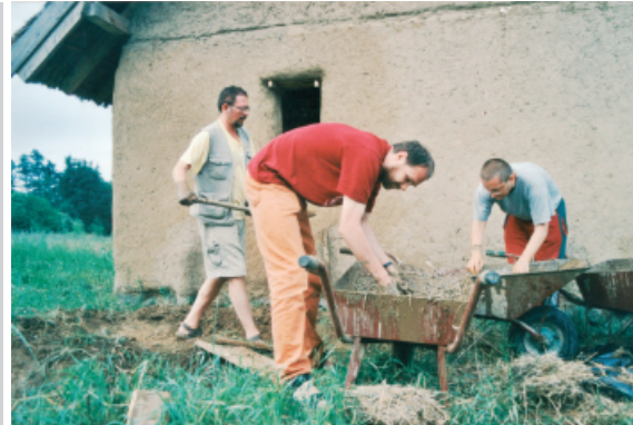
Figure 7. Construction of straw bale cottage; Photo Paulina Wojciechowska
