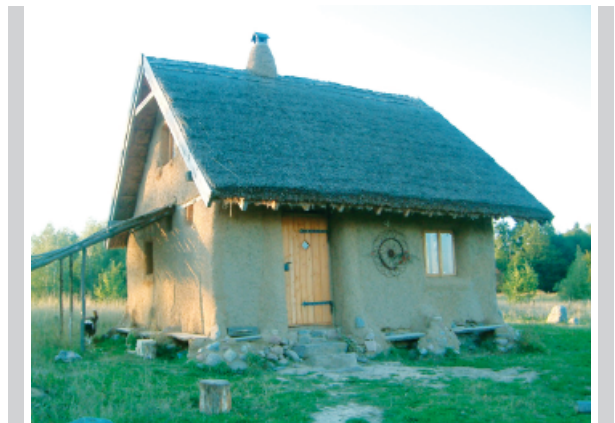
Figure 6. Cottage in Przelomka by Paulina Wojciechowska. First Straw bale construction in Poland; Photo Paulina Wojciechowska
