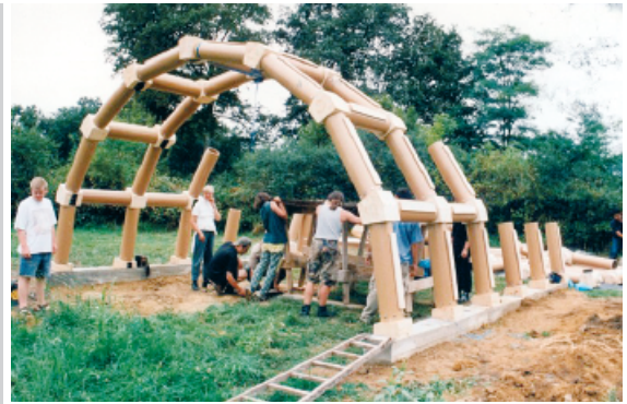
Figure 5. Paper tube construction by Shigeru Ban (Vitra Design Museum Workshop at the Domaine de Boisbuchet); Photo: author
