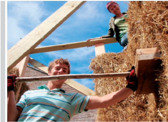
Figure 2. Construction of Straw Bales Bungalow retrofitting in Bridport, UK; Photo: author
