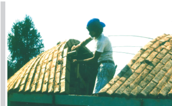
Figure 4. Nubian vault construction designed by Gernot Minke; photo: Gernot Minke
