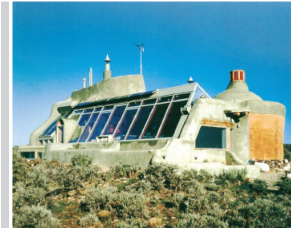
Figure 3. Earthship by Mike Reynolds in Taos, USA; Photo: Mike Reynolds
